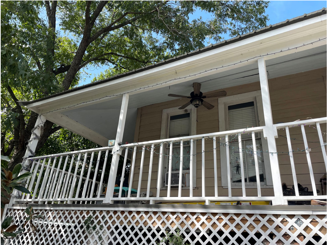
Photo 9: East elevation portion of the wrap around porch with non-original columns fronting West Street. Photo by HOP staff member, Cara Quigley, October 6, 2023.
